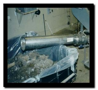
Another useful option on the press is a bagger. This device is placed at the exit of the discharge chute and catches all the compacted screenings. The bagger also seals in any odour and provides an alternative way to simply remove the screenings in a plastic bag instead of using a large heavy dumpster.
